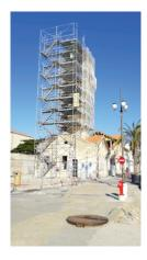
The lighthouse has deteriorated over time. That's why the commune of Grau du Roi began its restoration in 2016. Foundations, floors, facades, floorboards, roof, stairs, beacon, ladders... everything was inspected, then repaired or replaced!
